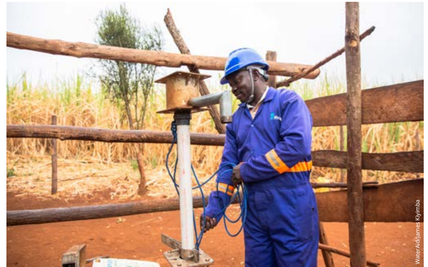
Stewart Kahumuza, hand pump mechanic, servicing the Kijenga village hand pump, Masindi district, Uganda. March 2025.
