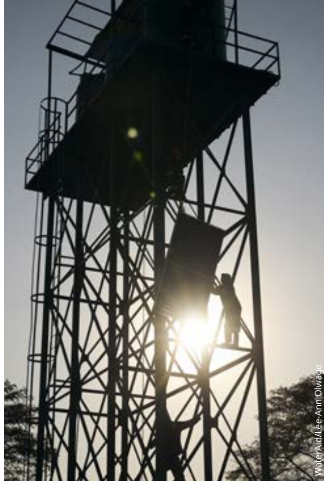
Solar panels being installed along with three new 10,000l water towers that will provide clean water to Sylvia Masebo community, Lusaka, Zambia. July 2025.
